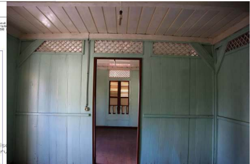
(wooden partitions with stiffener at mid-height)
