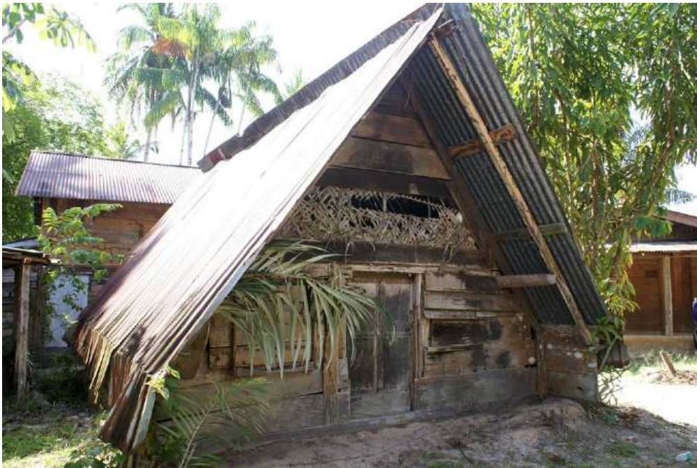
Before (with low door and vegetal ventilation "kopo")
