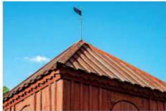
Roof boards at Bell tower Pēterā Street, photo: Krists Spruksts, 2020
