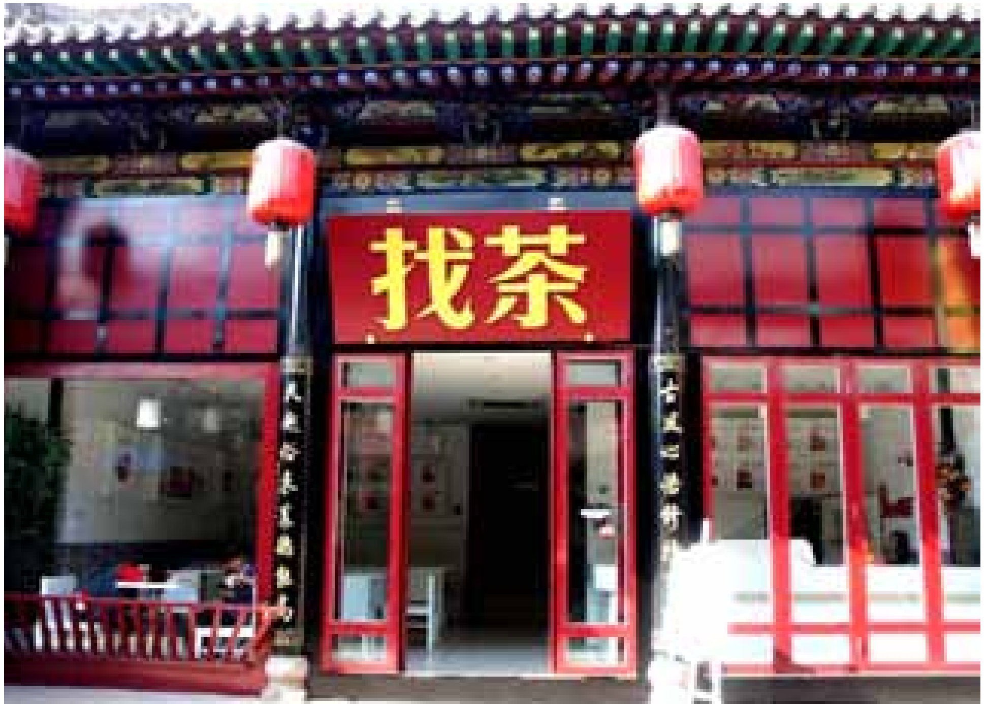
New buildings with odd facades
