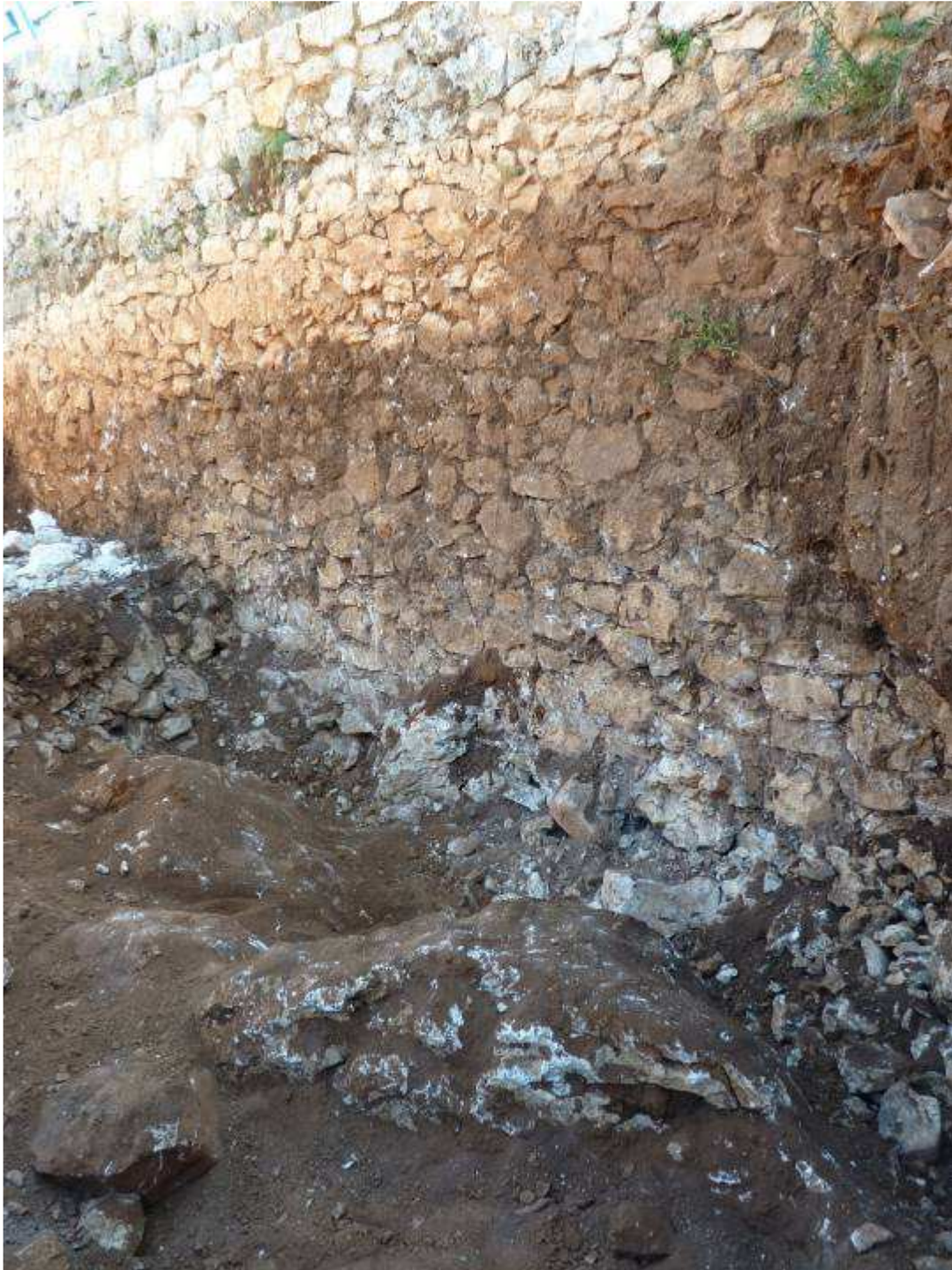
Pasha's tabija, works in progress, 2013
