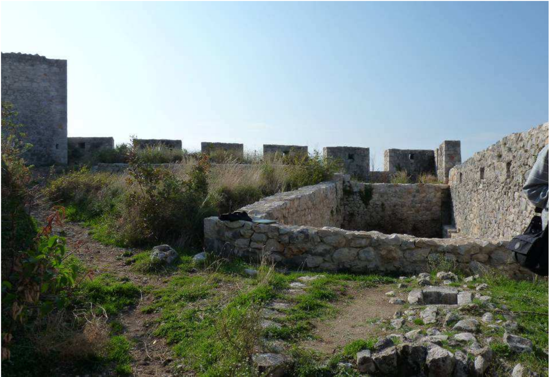
Pasha's tabija, condition before the works, 2012
