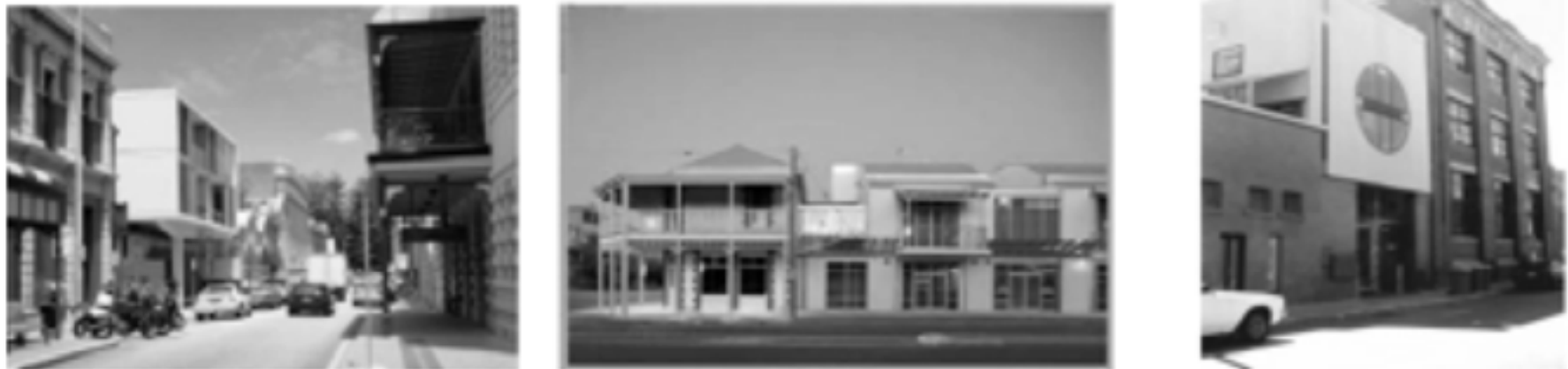
Figure 4b: examples of infill developments complying with the acceptable degree of deformation according to the Code (photos Agnieszka Kiera)
