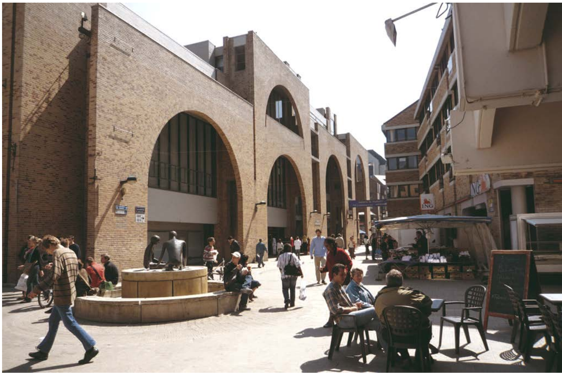
Upper entrance of railway station building along the pedestrian spine (rue des Wallons) and starting point of the platform.
